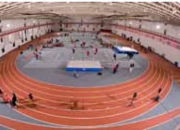
Fifty-foot-tall, 12-foot-wide precast panels form walls of the inner track and field area.
